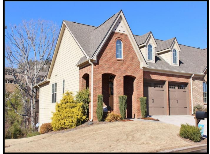
End Unit In City of Dahlonega
