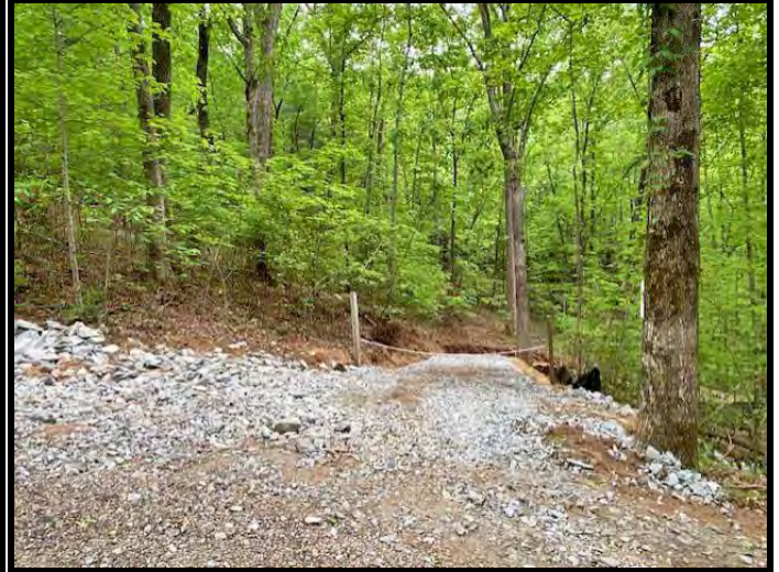
New Driveway Leads Into The Property
