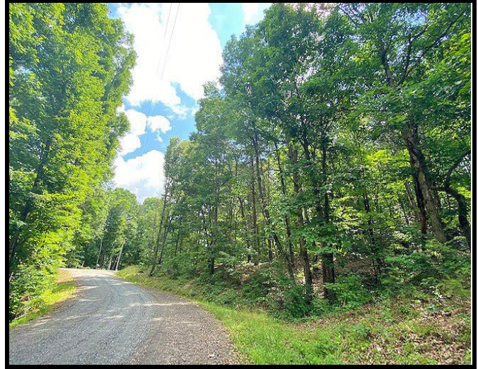
County Maintained Gravel Roadway
