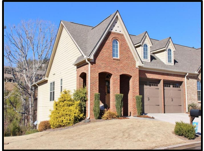
End Unit In City of Dahlonega
